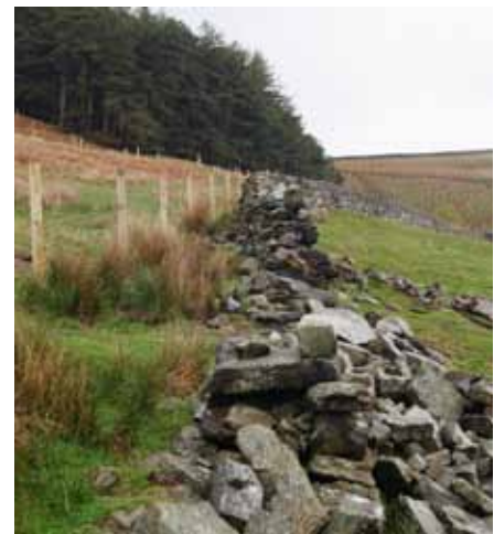
The estate has rebuilt over 1km of fallen wall
